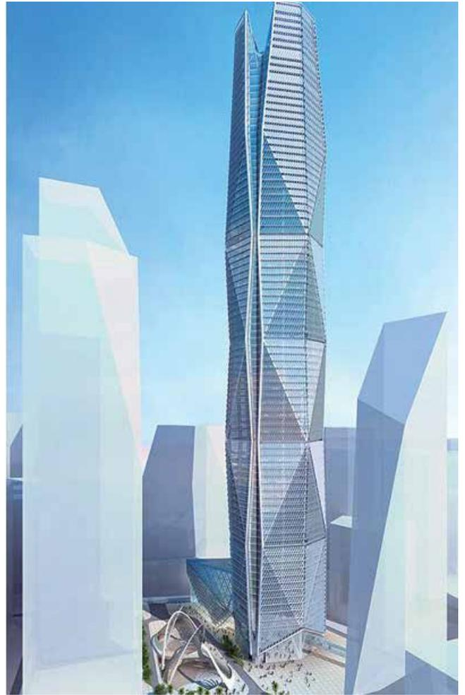
and perforated panels provides shade, amplifying the thermal efficiency of the triple-pane, and unitized glazing. Together, these shading devices minimize solar gain and internal cooling loads, reducing HVAC requirements. Electrical energy is reclaimed through a photovoltaic array installation on the tower's roof.
