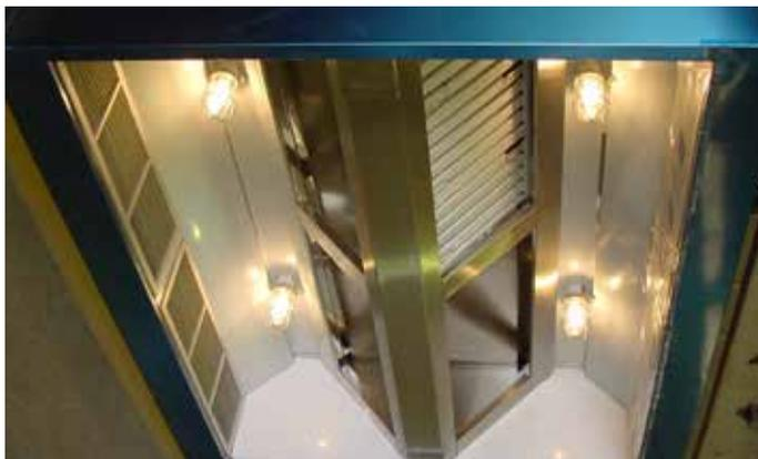
It is a known fact that the heated surface of cooking equipment convects heat to air around. As this air warms up, the air density decreases and becomes lighter than the surrounding. The lighter air creates an upward thermal current known as convection flow. The convection flow takes up the contaminants that are released during the cooking process and the surrounding air replaces the void created by the thermal current as illustrated in Figure 1
